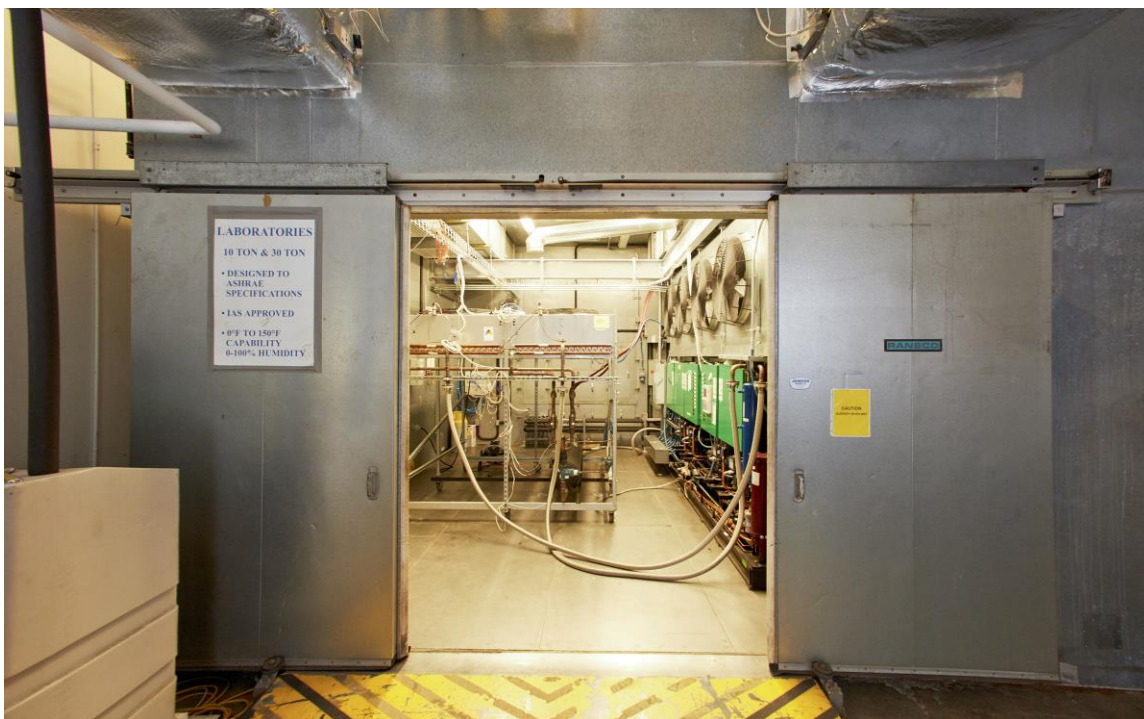
Figure 3. ORNL's large environmental chambers - outdoor chamber.
