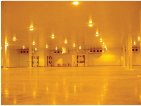
image 9: Inside the ASDA Distribution Centre source: Star Refrigeration (2003)
