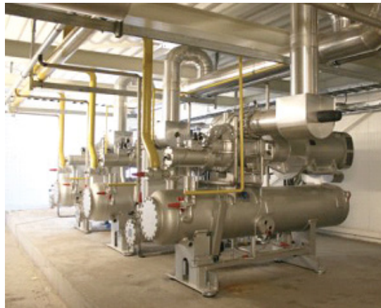
image 6: Three SAB193L compressors produce the refrigeration at Zellik
