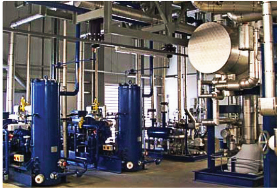
image 8: Inside the machinery room of ASDA's Lutterworth Distribution Centre
