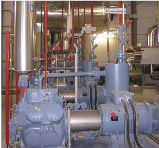
image 7: GEA Grasso 65HP compressors with variable-speed drive motors for optimised operation under partial load
