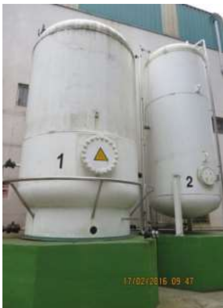
Storage facility R22 (37,000 kg)
