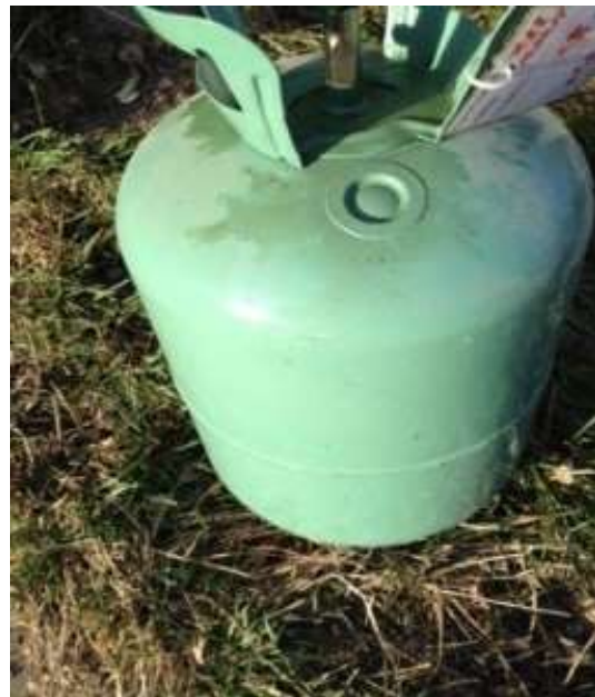
Unlabelled refrigerant cylinders containing R22
